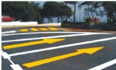
Parking Lot marking Victoria Island Lagos
