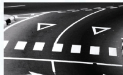
Hazard Teeth Markings Ojuelegba, Lagos
